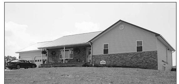
This 3,220 square foot Touchstone Energy Home owned by Daniel Hedinger has a guaranteed heating cost not to exceed $300, cooling not to exceed $191.
